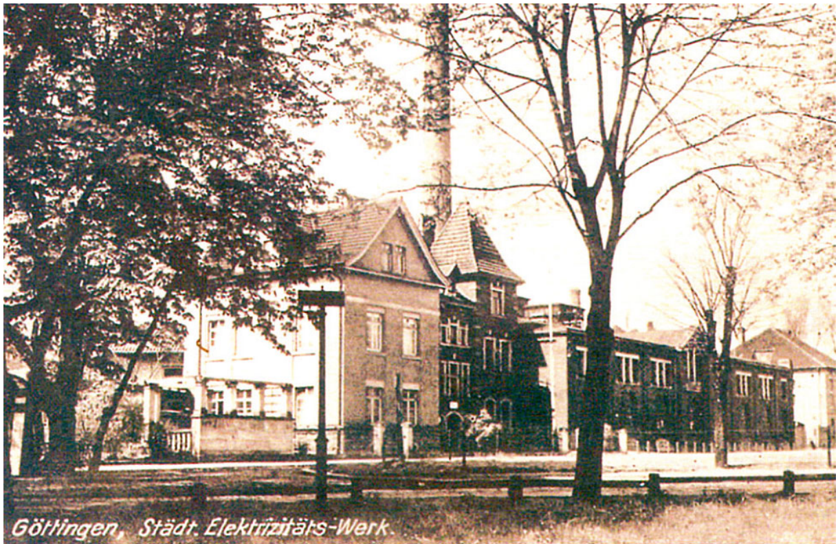
From 1899 on the grid: the power station at the train station.
